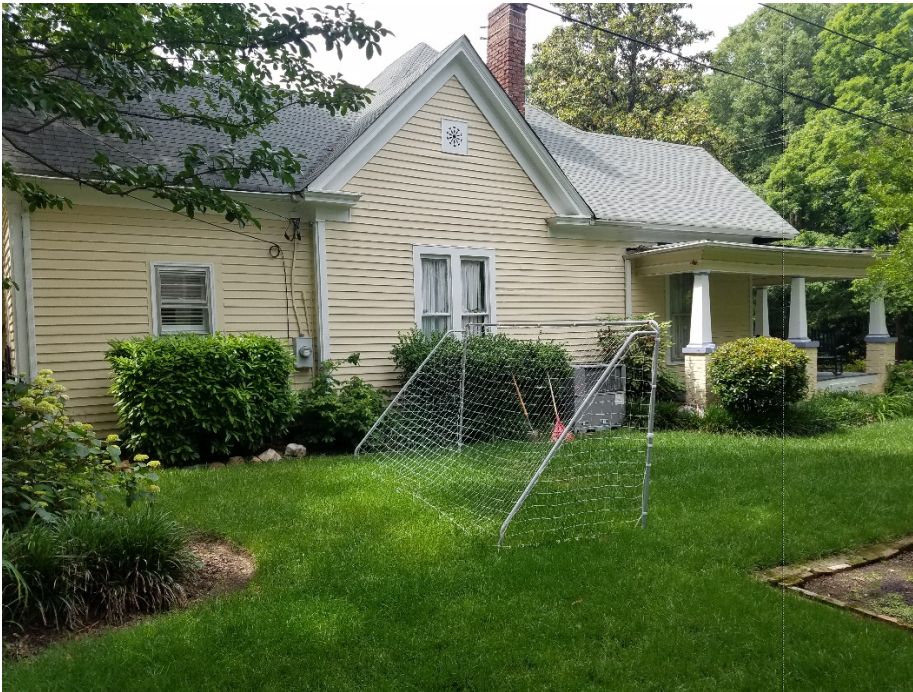
Existing Left (viewed from front) gable. Vent to be replaced with 36"x36" casement window.
