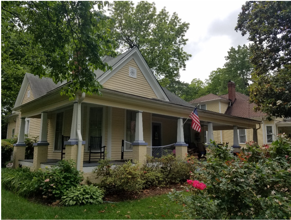
Existing View from Street
